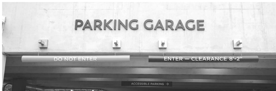
Figure. 2.2 Height clearance bar and height limits
