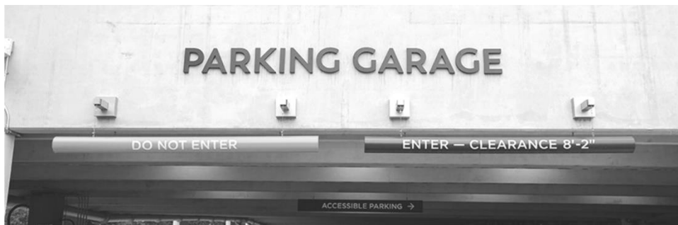
Figure. 2.2 Height clearance bar and height limits
