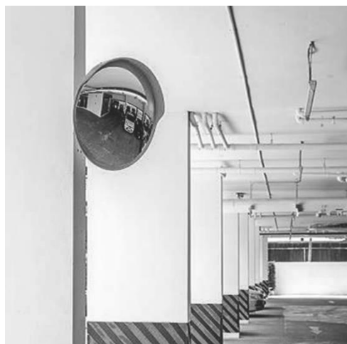
Figure. 2.3 Convex mirror can be provided at corners and blind spot areas to provide better visibility for motorists and pedestrian.
