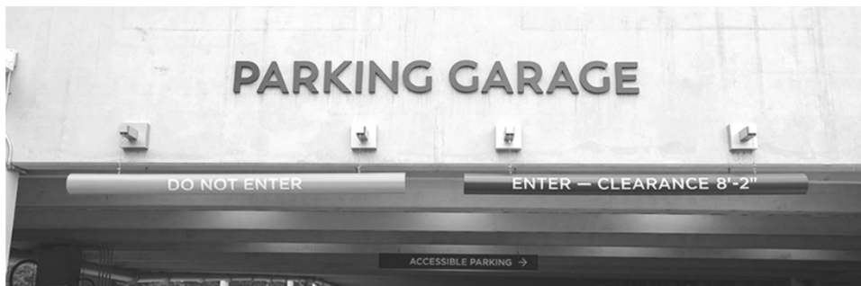
Figure. 2.2 Height clearance bar and height limits
